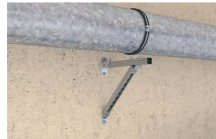
Spiral airduct on cantilever
