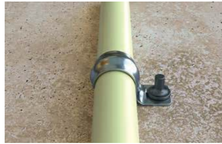
Fixing armoured conduits
