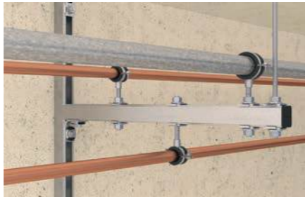
Cantilever construction with channel
