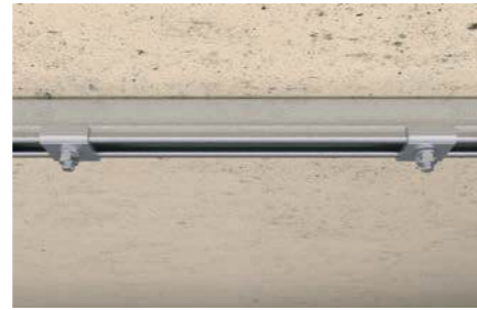
Channel installation at ceiling
