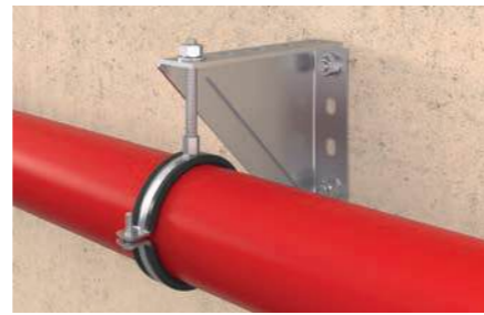
Heavy drainage pipe under angle bracket
