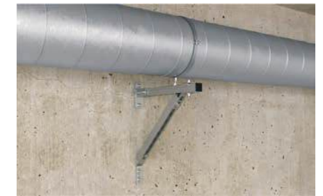
Spiral airduct on cantilever
