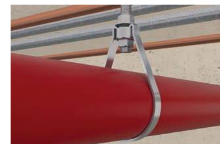
Sprinkler pipe installation
