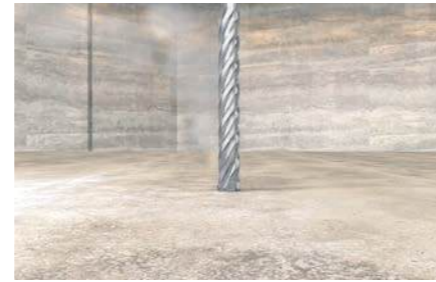
Drilling in floor plate
