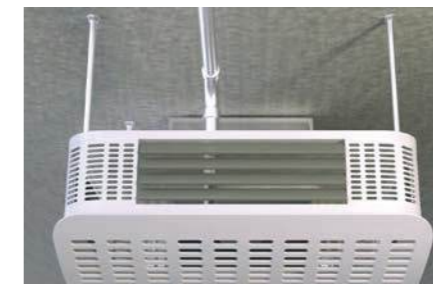
Suspended air-conditioners
