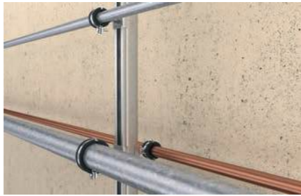
Lateral pipe mounting at channel
