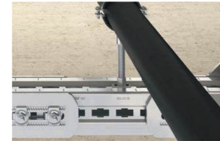
Installation of pipe clamps
