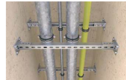
Pipe installation in escape route
