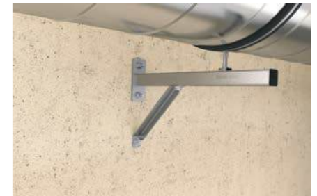
Ventilating pipe fixing at the wall
