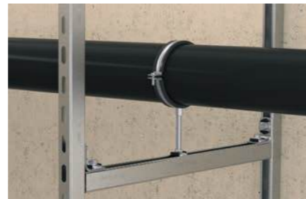
Pipe fixing on frame construction
