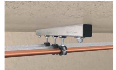
Pipe fixing at mounting channel
