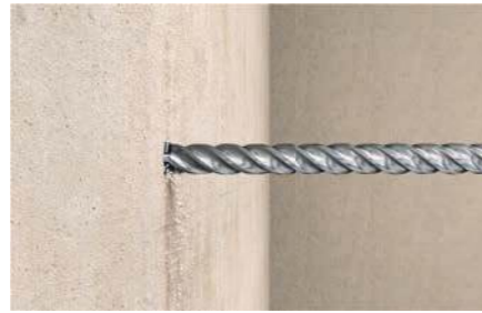
Drilling in concrete wall
