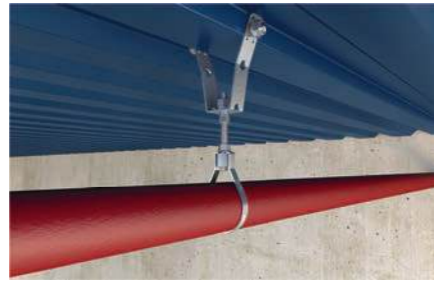
Sprinkler pipe installation to trapezoidal metal sheet
