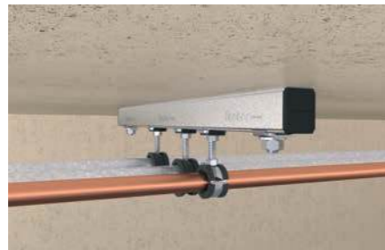
Pipe fixing at mounting channel
