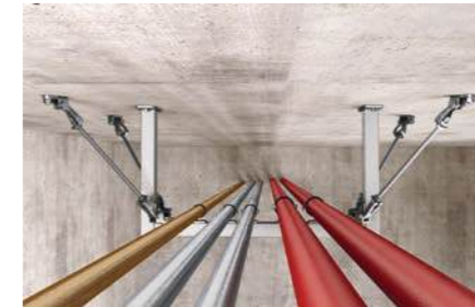
Bracing of frame construction with threaded rods
