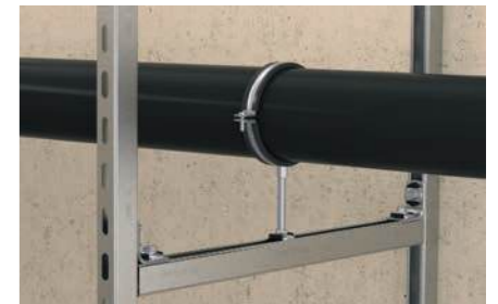
Pipe fixing on frame construction
