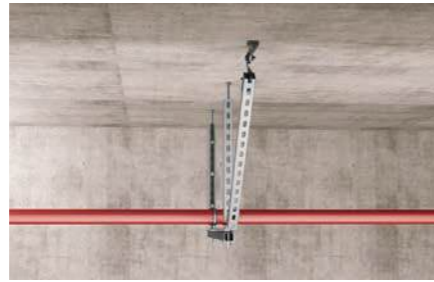
Rod stiffening for vertical seismic support
