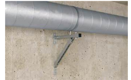
Spiral airduct on cantilever
