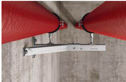
Bracing of cantilever construction
