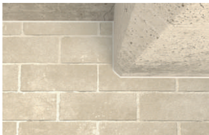
Construction joint application
