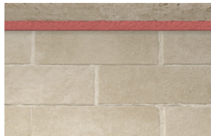
Construction joint application
