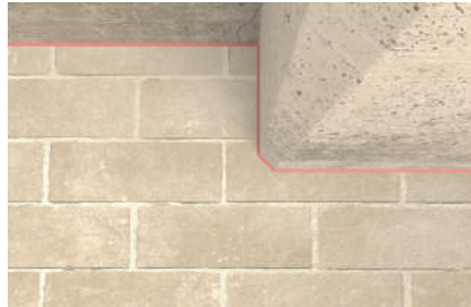
Construction joint application
