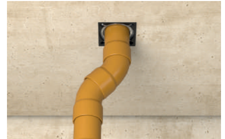
Installed pipe through FCID Plus device
