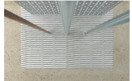
Mixed penetration through the wall
