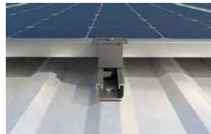
Roof with trapezoidal metal sheets covering
