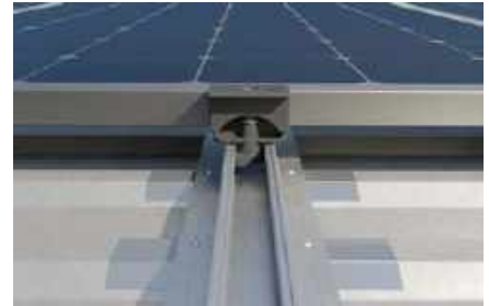
Roof with trapezoidal metal sheets covering
