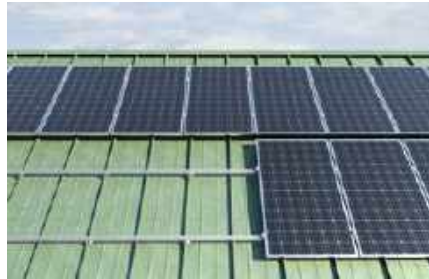
Pitched roof with flat standing seam covering
