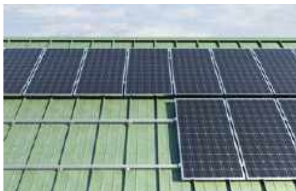
Pitched roof with standing seam covering
