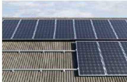
Pitched roof with corrugated sheets covering
