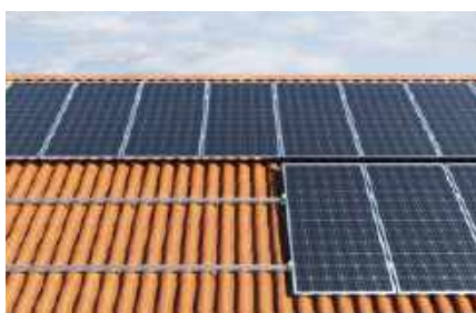
Pitched roof with tiles
