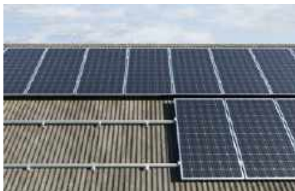
Pitched roof with corrugated sheets covering
