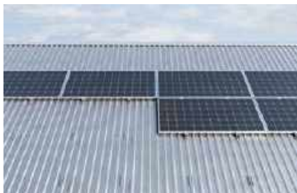
Roof with trapezoidal metal sheets covering
