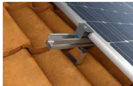
Pitched roof with tiles
