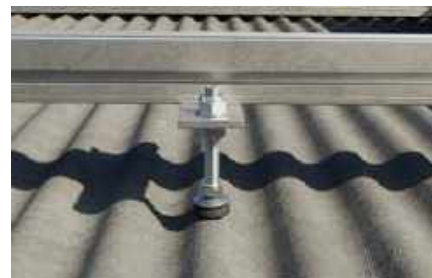
Pitched roof with corrugated sheets covering
