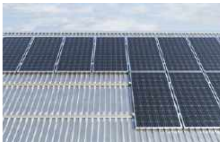
Roof with trapezoidal metal sheets covering
