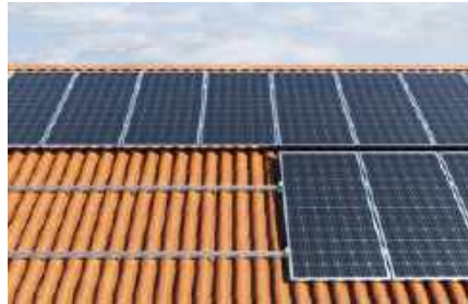
Pitched roof with tiles
