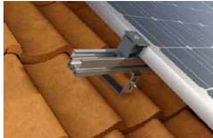
Pitched roof with tiles
