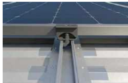
Roof with trapezoidal metal sheets covering
