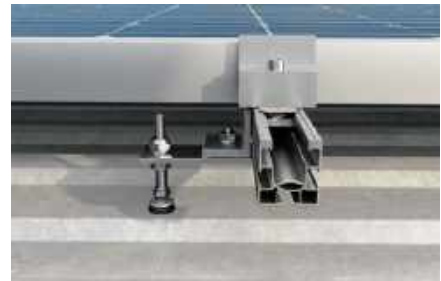
Roof with trapezoidal metal sheet covering
