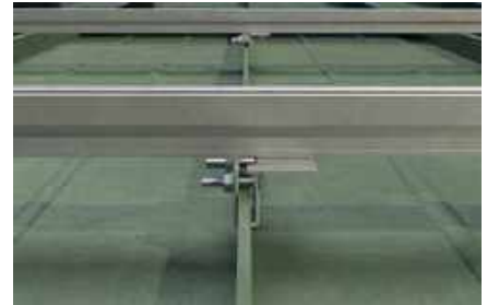
Pitched roof with flat standing seam covering
