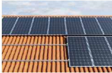
Pitched roof with tiles
