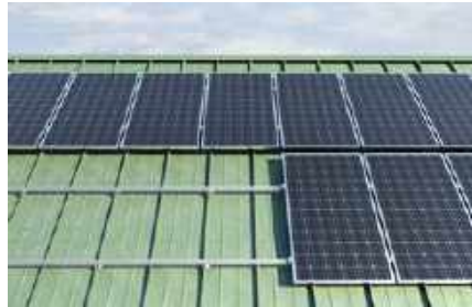
Pitched roof with standing seam covering
