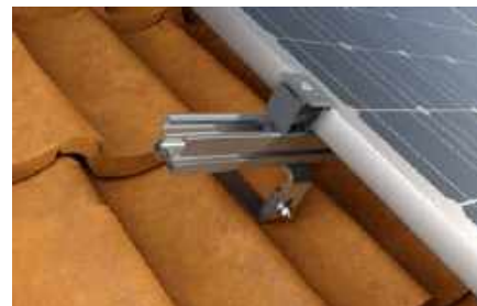
Pitched roof with tiles
