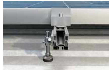
Roof with trapezoidal metal sheet covering
