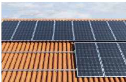
Pitched roof with tiles
