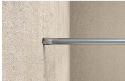
Hollow drilling in concrete
