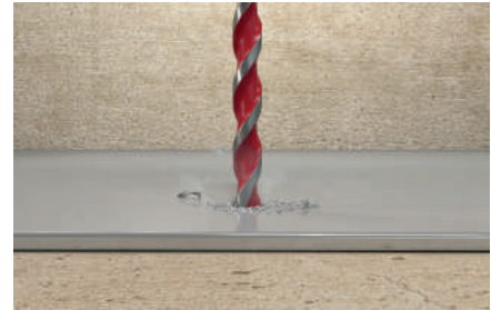
Drilling the material combination of metal and concrete
