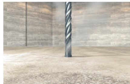
Drilling in floor plate
