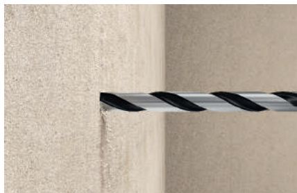
Drilling in concrete
