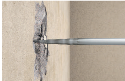
Chiseling in concrete wall
