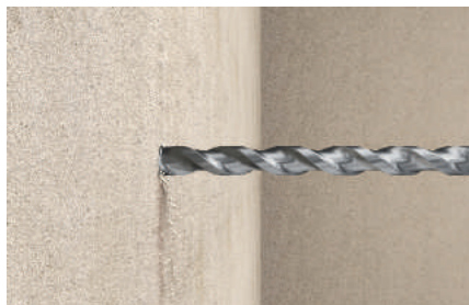
Drilling in concrete wall
