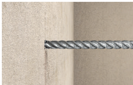
Drilling in concrete wall
