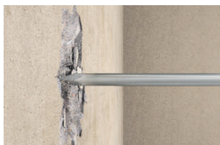
Chiseling in concrete wall
