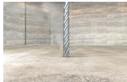
Drilling in floor plate
