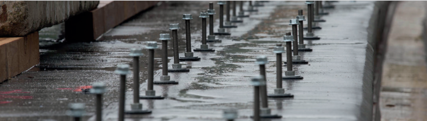
Bridge edge beam fixing
